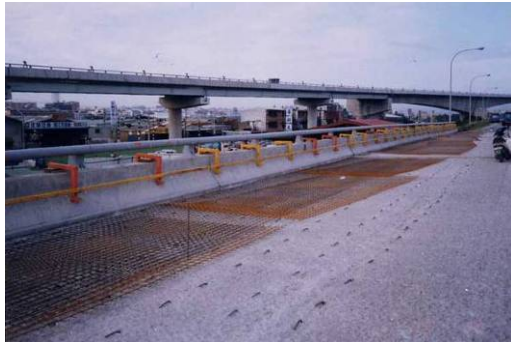
(c) 橋面版刨除面植筋
