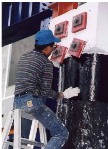
(g) CFRP 貼片貼附
