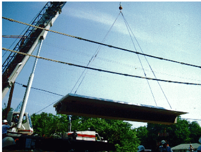
(c) 吊車組裝作業
