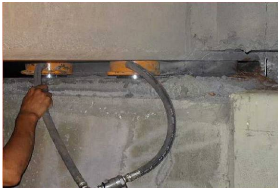
(a) 扁平式千斤頂置換橡膠支承墊
