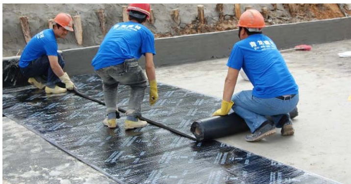
防水層 ( Waterproofing membrane )
